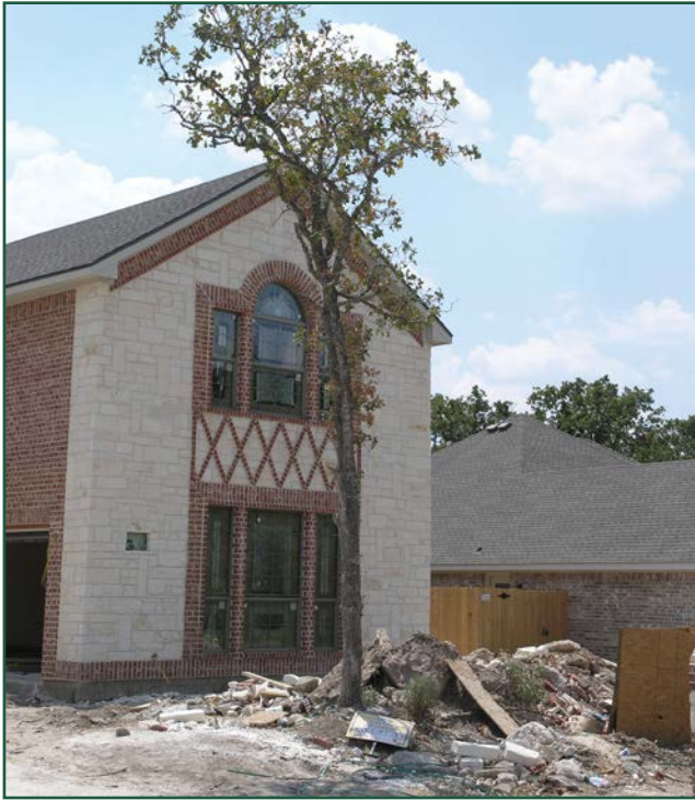
Figure 2. Mechanical damage, root disturbance, soil compaction, and other stress factors resulting from the urbanization of post oak woodlands. Source: David N. Appel
